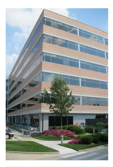
Flexibility in architectural design is illustrated in this 300,000 sq. ft. office building in Waltham, Massachusettes. The use of precast concrete elements add a level of contrast and detail to the brick and glass elements of the exterior envelope.
