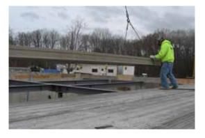
This four story, 150 bed residence hall is home to first year students. Completed in 2004, Strescon fabricated and installed 41,000 sf of both 8" and 10" thick Strescore plank. The plank ceilings were finished with a textured sprayed on paint providing a pleasing bright finish.
