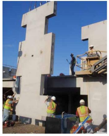
After the precast concrete componets were erected, the structural steel framed health care facility was constructed on top of the garage structure.
