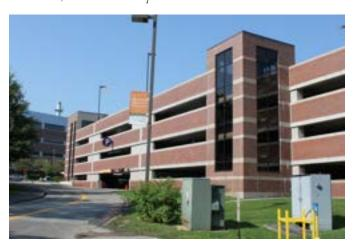
Architects: **Desman Associates -** Boston, MA Construction Manager: **Harvey Construction Corp.** Bedford, NH The all-precast concrete parking structure, part of the Exeter Hospital campus in Exeter, New Hampshire, features precast concrete double tees, columns, beams, wall panels and spandrel panels from Strescon Limited (Saint John, New Brunswick and Bedford, Nova Scotia).
