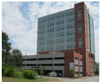
This unique project features a 6 story medical office building sitting atop a 4 level 139,000 sf parking garage. Strescon Limited provided the total precast concrete garage which supported the office building on top of the garage columns.
